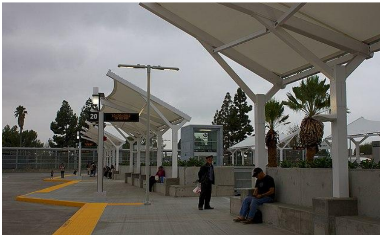
Figure 4. Above are photographs (from top to bottom) of the Azusa Downstation, City of
