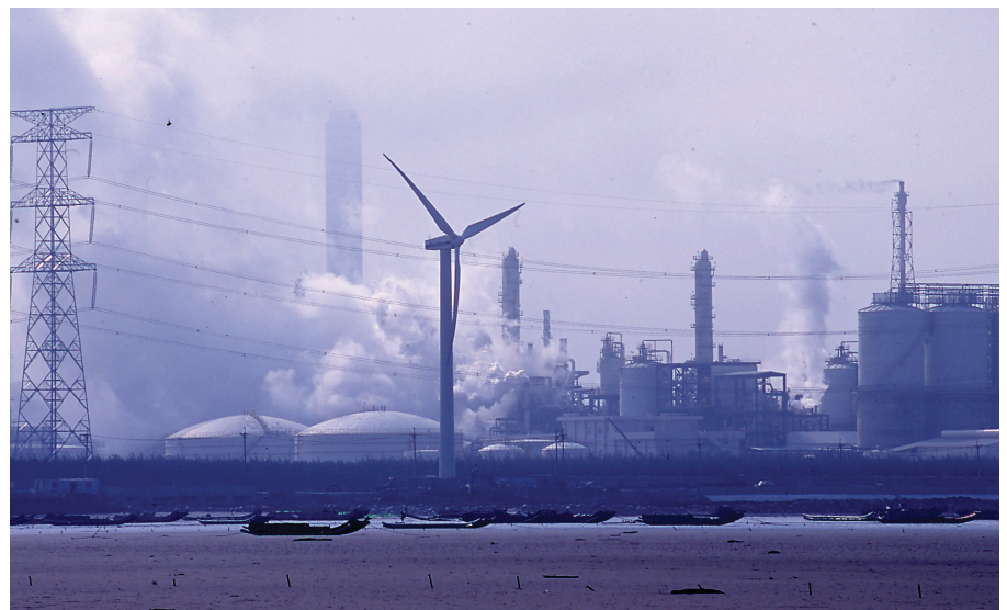
Figure 4. Sixth Naphtha Cracker Complex, January 2003.
