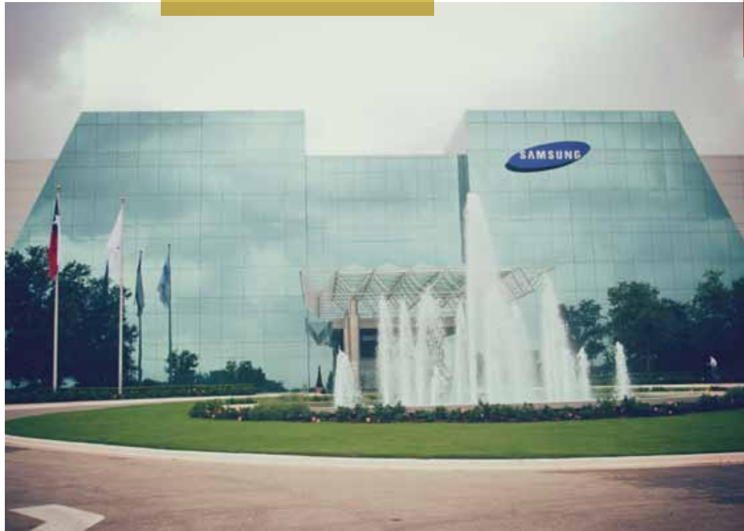
Mid- and large-size commercial customers can receive up to $200,000 in rebates from Austin Energy to make energy efficiency investments such as installing new HVAC equipment, reflective roofs, motors and variable frequency drives, and other improvements that help lower their energy bills.
