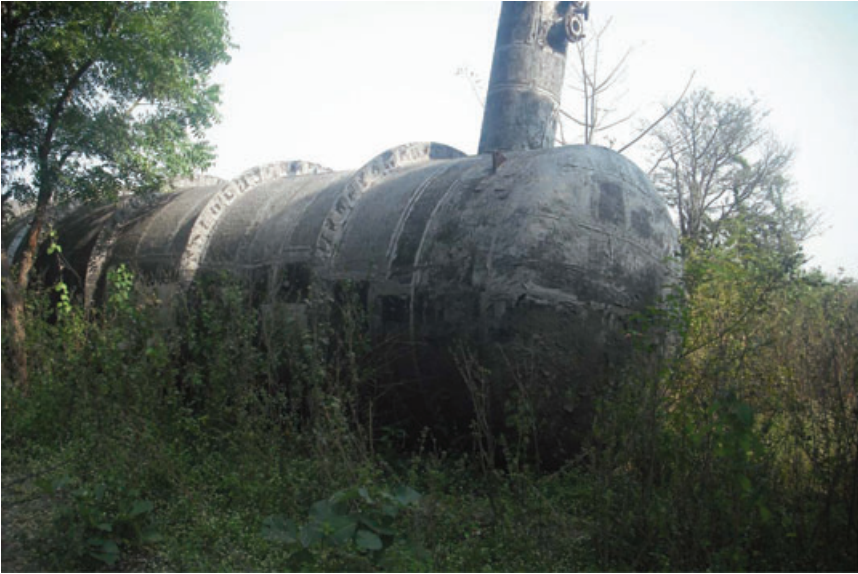
FIGURE 1. Tank 610 at the old Union Carbide plant in Bhopal India. Forty tons of toxic methyl isocyanate were released from this tank in the early morning hours of December 3, 1984.
