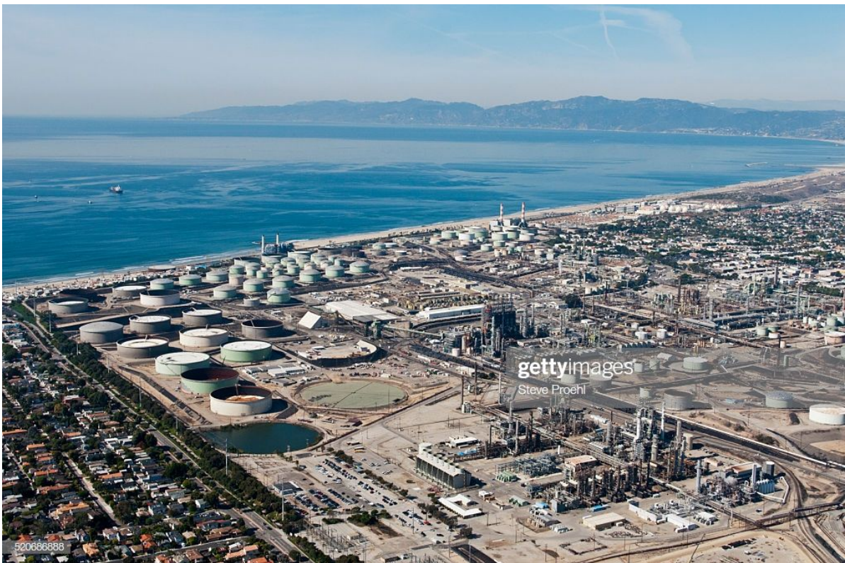
Fig 7: A photo of the Chevron refinery in El Segundo is shown right next to residents homes. Courtesy of Getty Images
