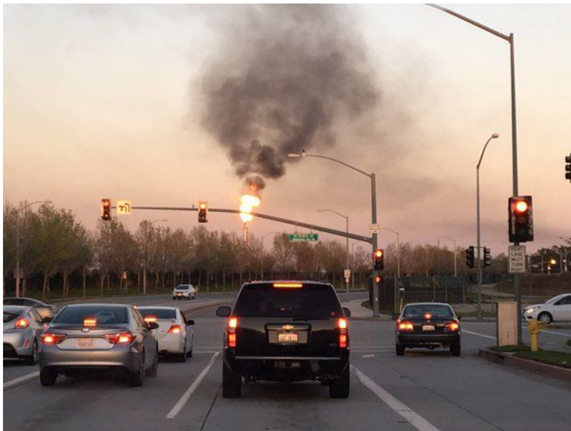
Fig 11: Power outage causes “flaring” burnoff at Torrance oil refinery, October 15th, 2016, Prima News accessed October 26th, 2019
