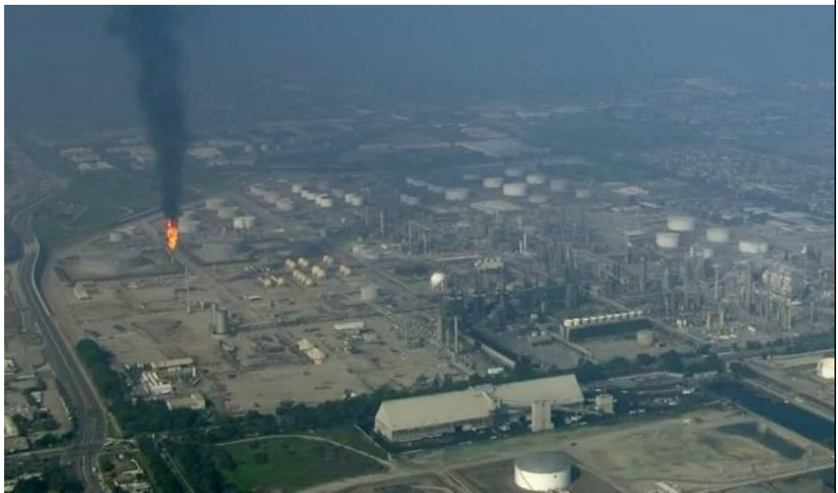
Fig 12: Kandel Jasont, ExxonMobil Refinery Explosion , February 18th, 2015, NBC Los Angeles accessed October 25th, 2019
