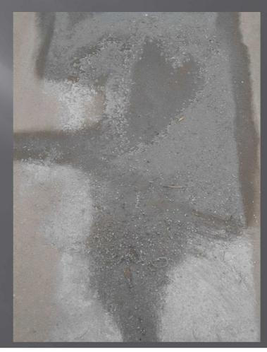
WEST OF THE BUILDING BEHIND THE PALLETS, PELLETS WERE OBSERVED COMING FROM INSIDE THE BUILDING THRU CRACKS IN THE OUTER WALL.
