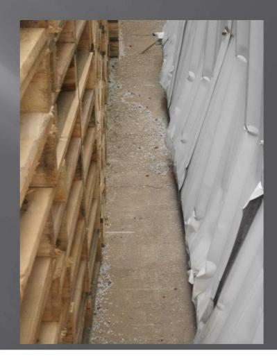
SIMILAR TO THE PREVIOUS SLIDE JUST FURTHER NORTH OF THE PALLETS, PELLETS WERE OBSERVED AROUND A CRACK IN THE OUTER WALL.
