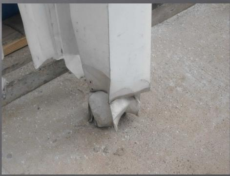
ON THE NORTH SIDE OF THE BUILDING AT THE DOOR. ATTEMPTS TO STOP THE PELLETS FROM TRAVELING OUT OF THE BUILDING HAVE BEEN MADE FROM INSIDE. HOWEVER THERE SEEMS TO BE A SMALL SPACE WHICH PELLETS ARE ABLE TO GET OUT FROM.
