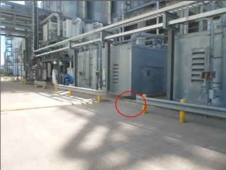
CLOSER IMAGE. NOTE THAT HOLES ON PAVEMENT DRAIN TO THE INTERNAL DITCH FOR PROCESS AREA. WATER FROM THIS DITCH IS DISCHARGE D INTO OUTFALL 009.
